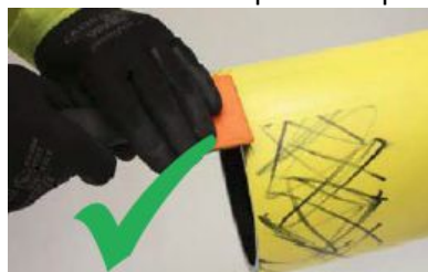
Figure D17 – Electrofusion
