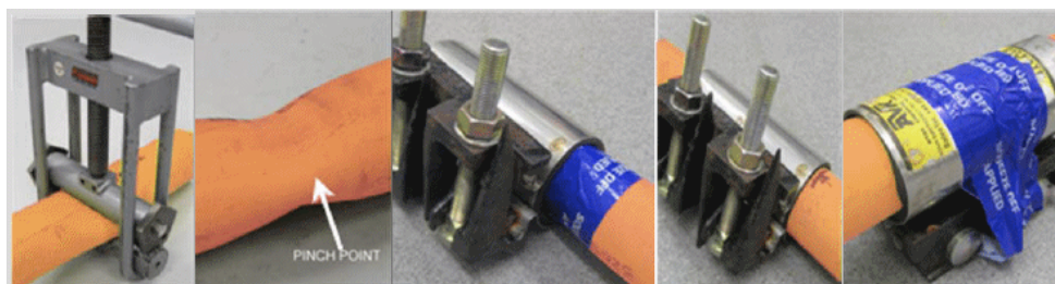
Figure 42- Fitting Mechanical Repair Clamp Over Squeeze-off Pinch Point
